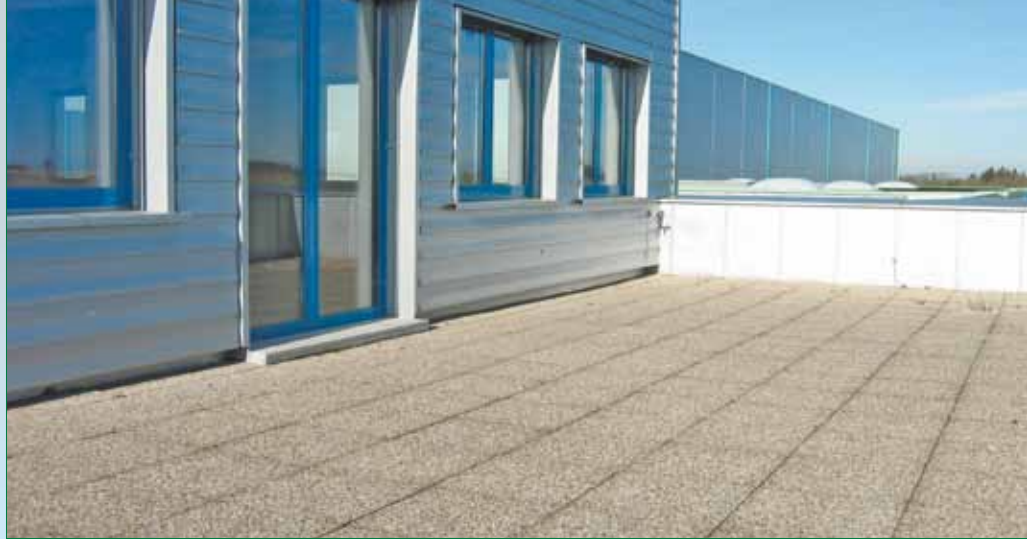
terrace with AUSTROPLAN sealed with roof liners and laid out with concrete plates
