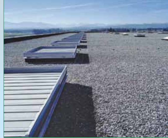
gravel ballast roof systems
