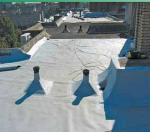
bonded roof system with AUSTROPLAN FG+V
