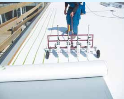
applying the roof sheet adhesive
