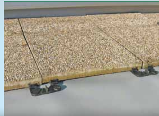
terrace with AUSTROPLAN sealed with roof liners and laid out with concrete plates
