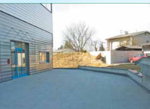
lining of utility system with ballast
